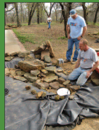
After the bucket that contains the pump was settled into place, much of the hole was filled with cinder blocks and large rocks collected from our property.
