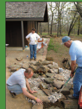
The pond liner edges were covered with large rocks, and decorative river rock was used to fill in the gaps. A garden hose soon filled the hole with water once this step was finished.
