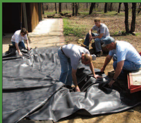
Rubber pond liner was placed in the hole and trimmed to size, leaving enough overlap around the edges to accommodate some rocks and hold it in place.
